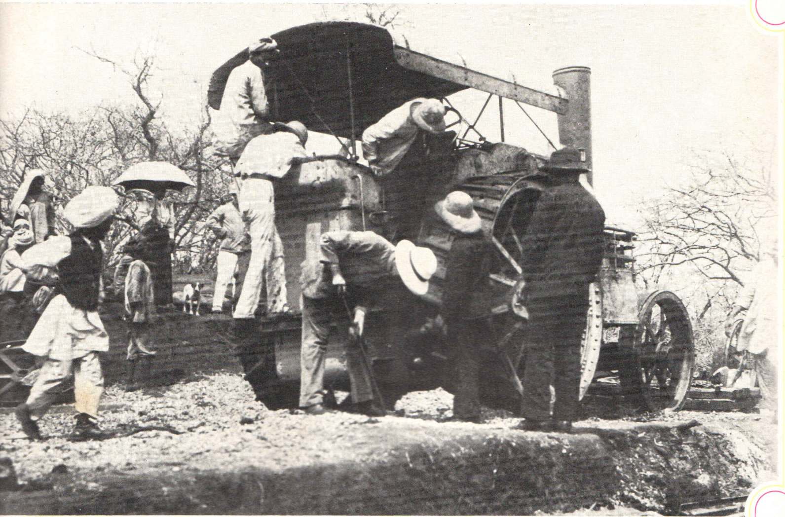
A traction-engine, one of the few large pieces of equipment used, proved an invaluable addition to coolie labour for hauling heavy loads and levelling rough surfaces.
