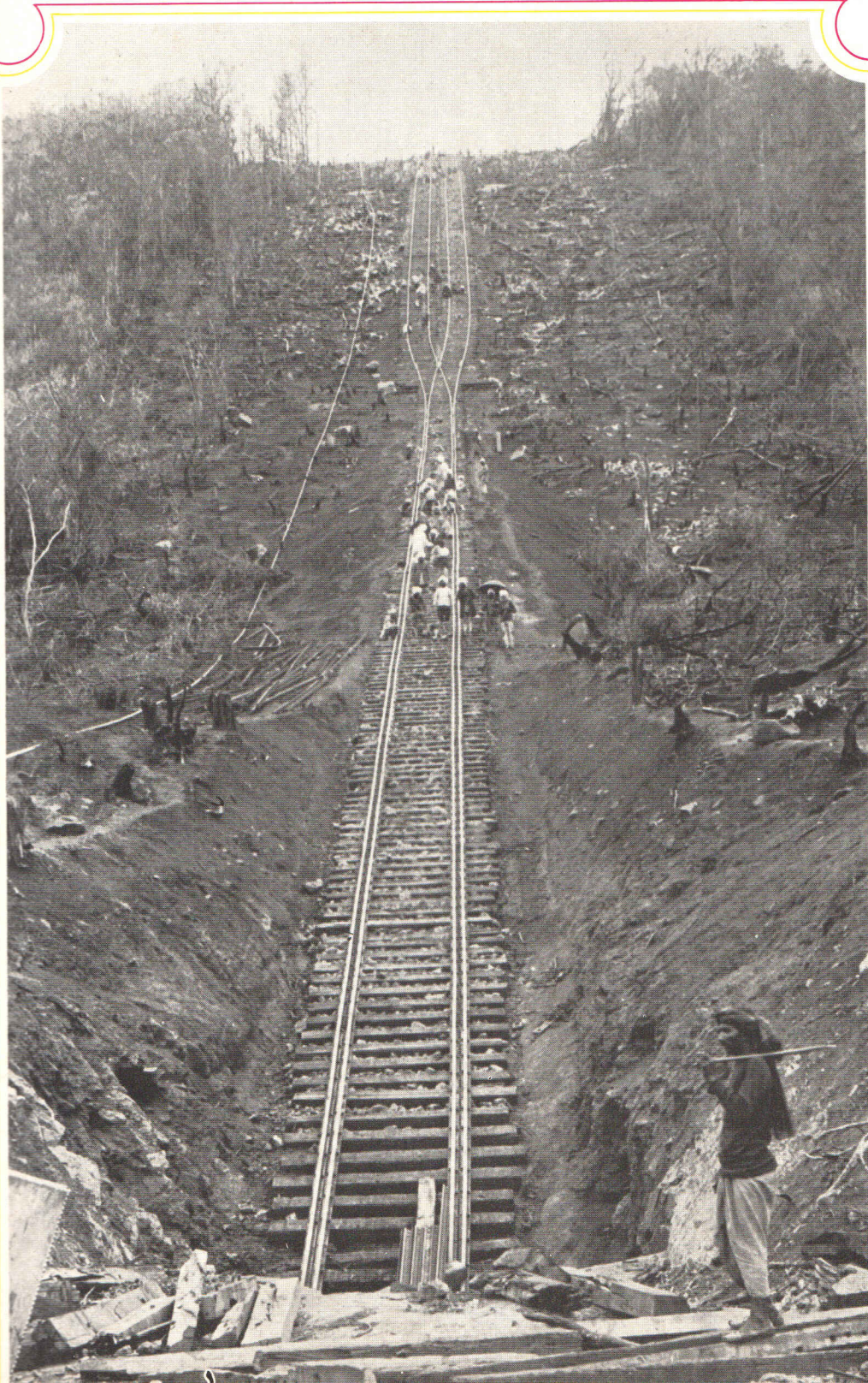
The angled platforms (above) that bore men and equipment up and down the 1,500-foot eastern wall of the Rift Valley (left) terminated at docking-bays so that the supply-wagons could run off on to level tracks.
